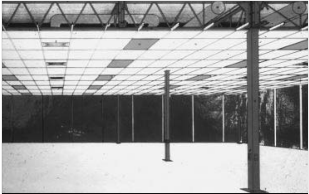
Fig. 7.39 IBM pilot head office, Cosham, UK, 1973; Foster Associates, architects; Anthony Hunt Associates, structural engineers. The structure was a steel framework with lightweight triangulated beam elements. These created a combined structural and services zone, at roof level which was essential to achieve the required flexibility in the use of the interior. (Photo: Anthony Hunt Associates)
