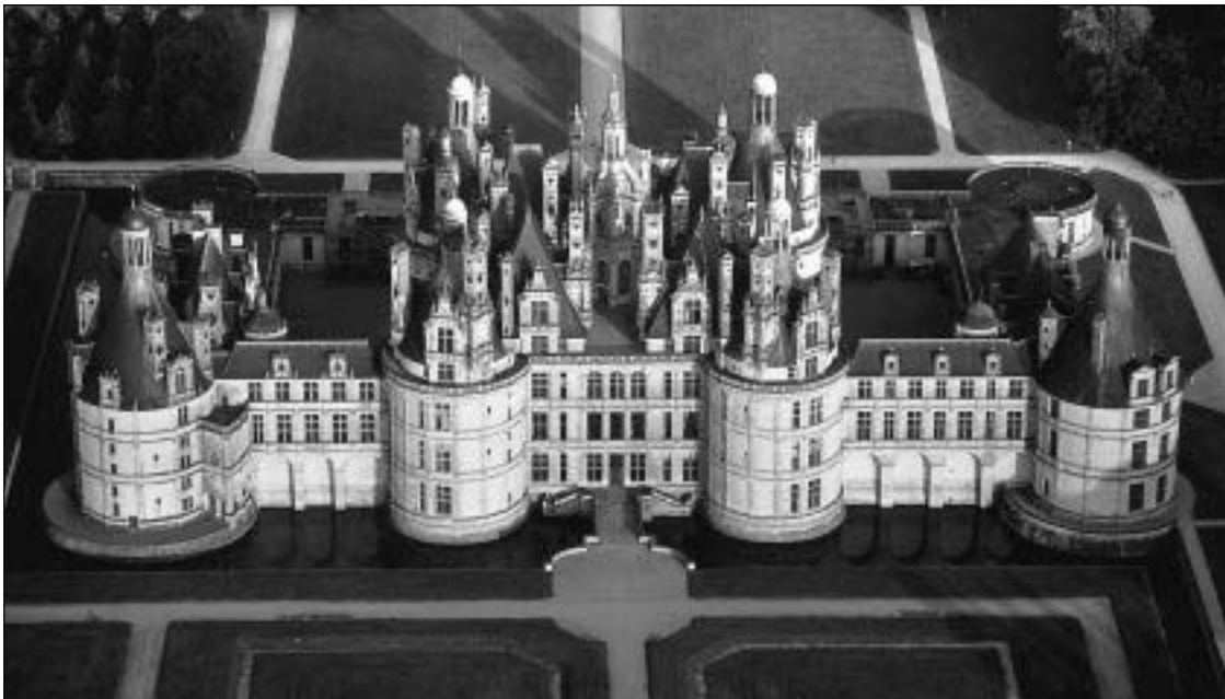
Fig. 1.12 Château de Chambord, France, 1519–47. One of the grandest domestic buildings in Europe, the Château de Chambord has a loadbearing masonry structure. Most of the walls are structural; the floors are either of timber or vaulted masonry and the roof structure is of timber. (Photo: P. & A. Macdonald)
