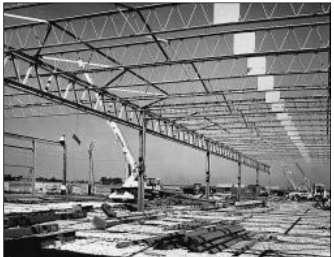
Fig. 5.16 Single-storey steel framework. Although some of the structural connections here are rigid, the majority of the horizontal elements have hinge joints. The regularity of the arrangement and the presence of a triangulated bracing girder in the horizontal plane (top left) are typical of a discontinuous framework. (Photo: Photo-Mayo Ltd)
