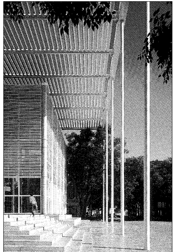
Fig. 1.6 Willis, Faber and Dumas Office, Ipswich, UK, 1974; Foster Associates, architects; Anthony Hunt Associates, structural engineers. The basic structure of this building is a series of reinforced concrete coffered slab floors supported on a grid of columns. The external walls are of glass and are non-structural. In the finished building the floor slabs are visible only at the perimeter. Elsewhere they are concealed by floor finishes and a false ceiling.
