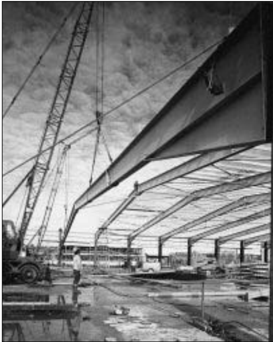
Fig. 5.20 The ubiquitous portal frame is a semi-form-active structure. The main elements in this example have 'improved' I-shaped cross-sections. (Photo: Conder)
