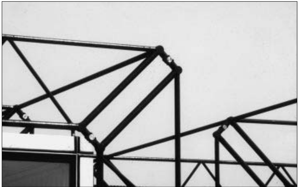
Fig. 7.28 Patera Building; Michael Hopkins, architect; Anthony Hunt Associates, structural engineers. The ingenious use of pin connections and cast nodes allowed a fully rigid joint to be made between the principal elements which could be easily assembled. (Photo: Anthony Hunt Associates)
