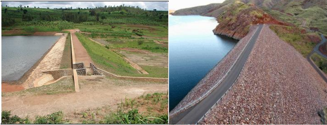
Figure7-: Sample of earth fill dam
