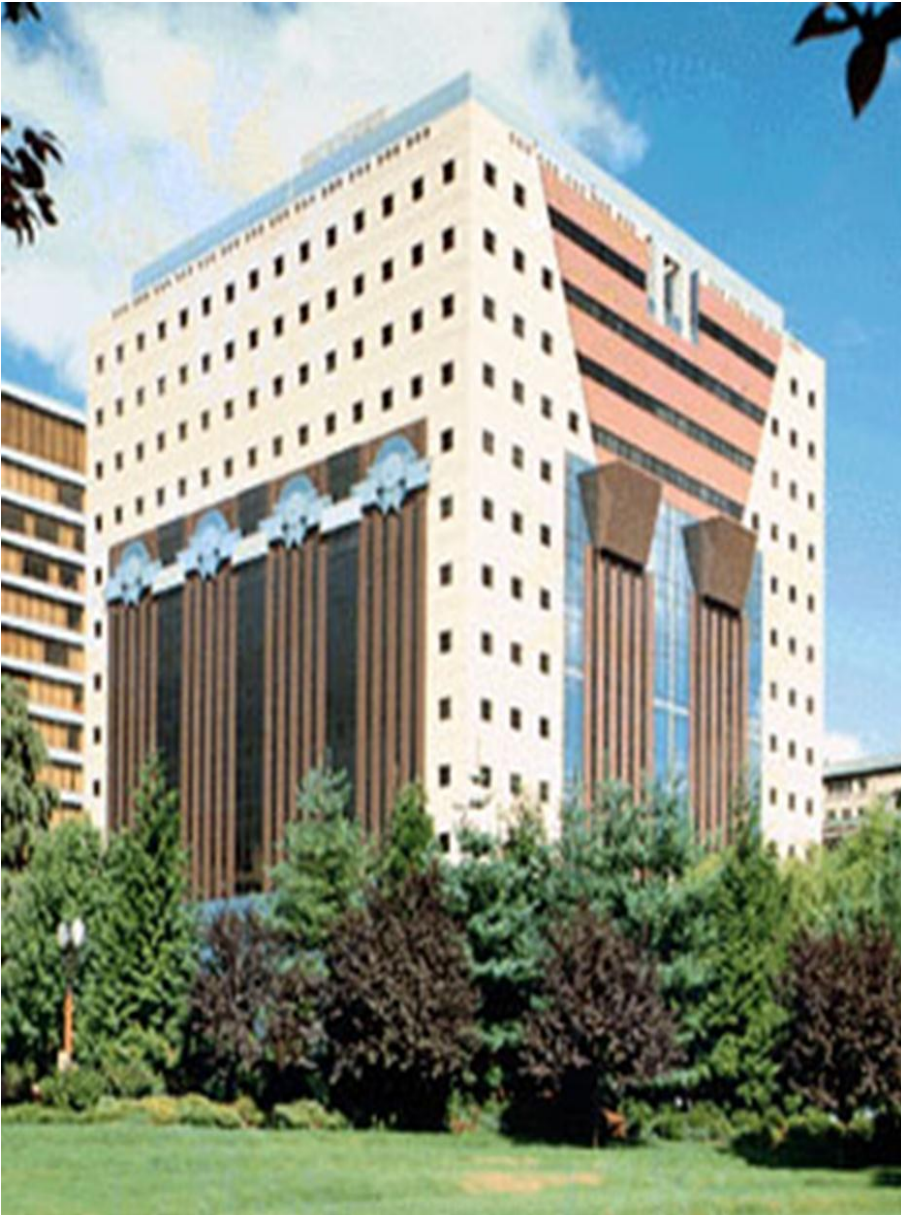
Portland Public Services Building, 1982. Michael Graves.
