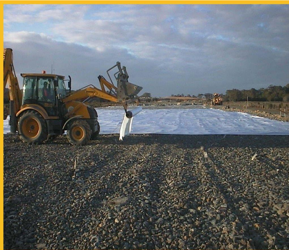
Geo-fabrics and Geo-synthetics used on Pacific Highway
