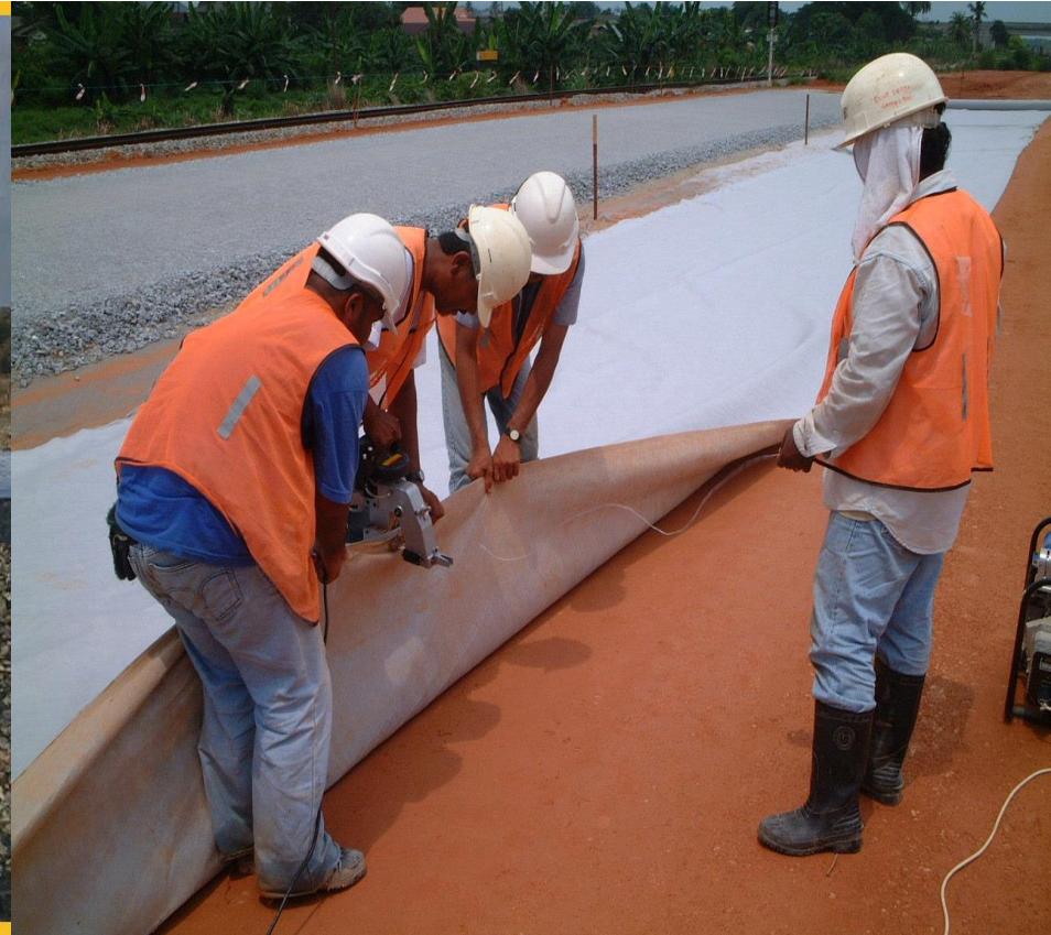
Geo-fabrics and Geo-synthetics used on Pacific Highway
