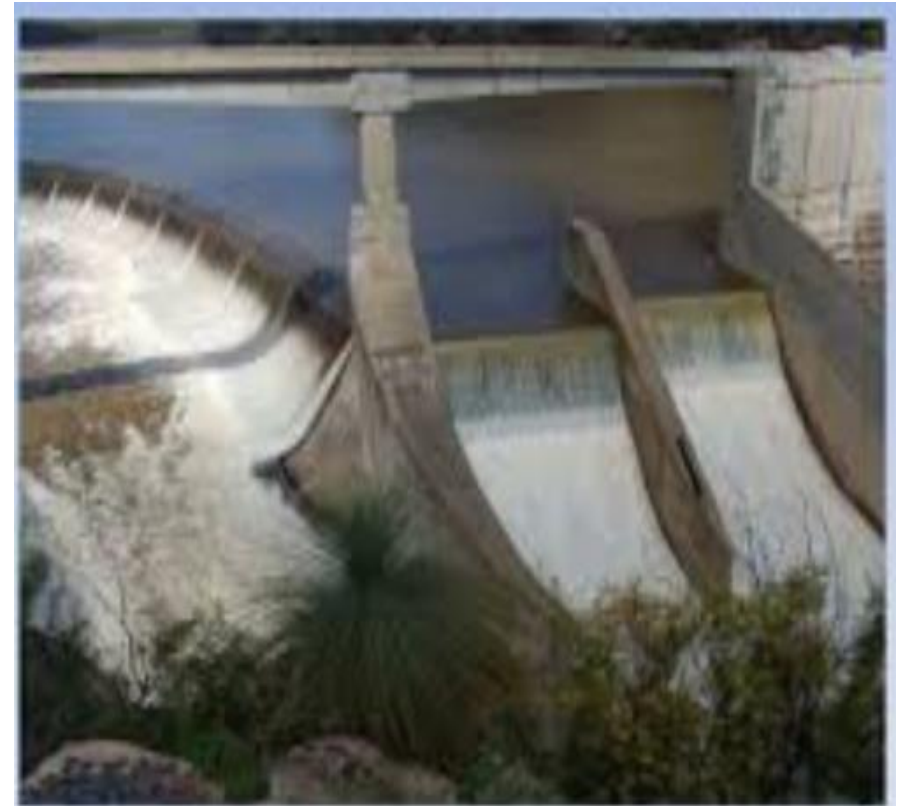
Figure 2.6-b: A typical side channel spillway
