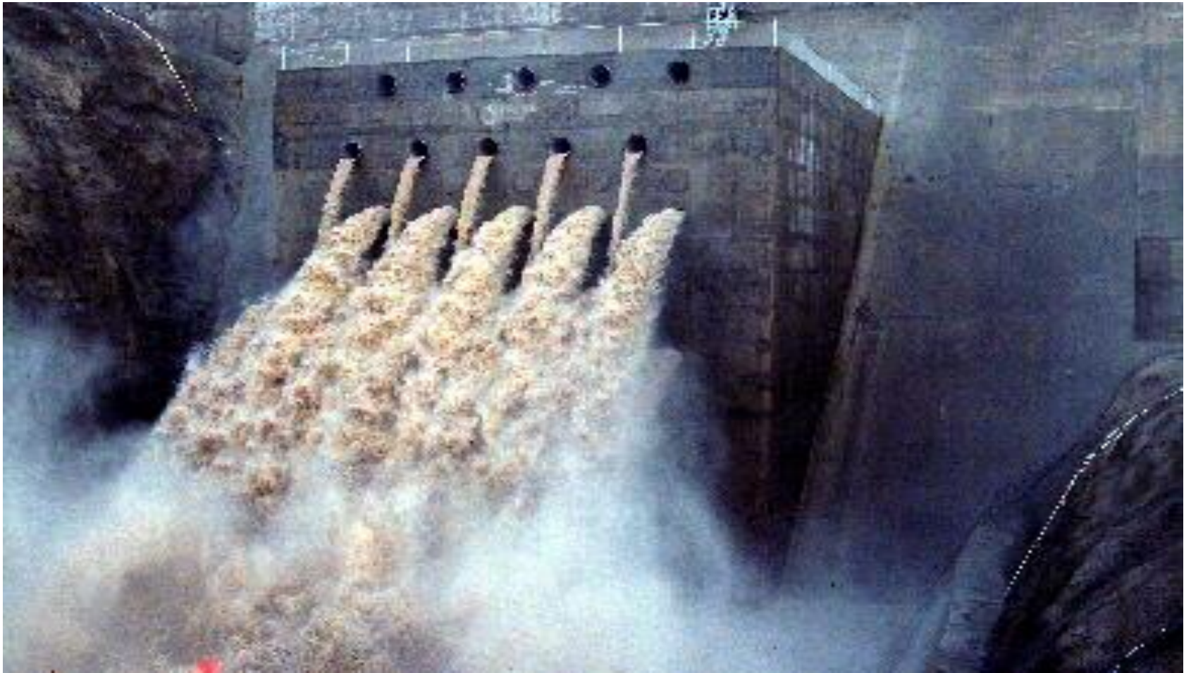
Figure 2.1: Free over fall or straight drop spillway
