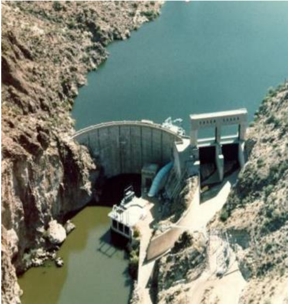
Figure 2.5: Chute Spillway
